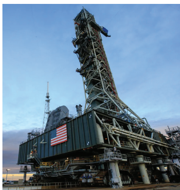
Launch pad ground support equipment
